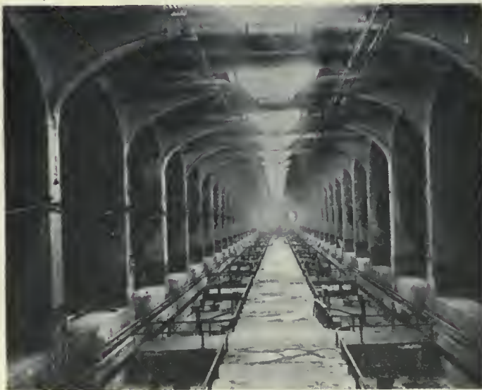
Fig. 8—Final Filter Gallery.
